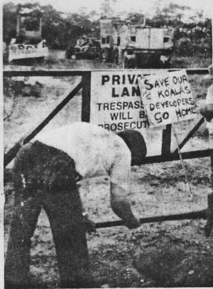
PETER Primrose plants a native tree in front of the bulldozers.
