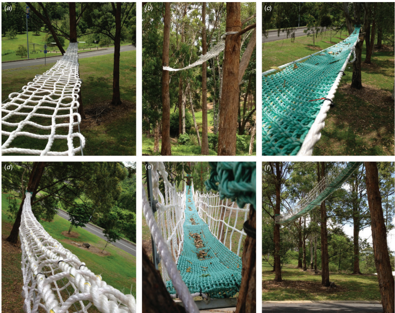
Fig. 1. The four different rope-bridge designs: (a) rope-ladder (45 cm wide), (b) ground view of the rope-ladder, (c) woven rope-mesh (34 cm wide), (d) rope-sausage (28 cm wide), (e) 3-sided rope-bridge (51 cm wide), and (f) ground view of the 3-sided rope-bridge. Photographs by B. Taylor.
